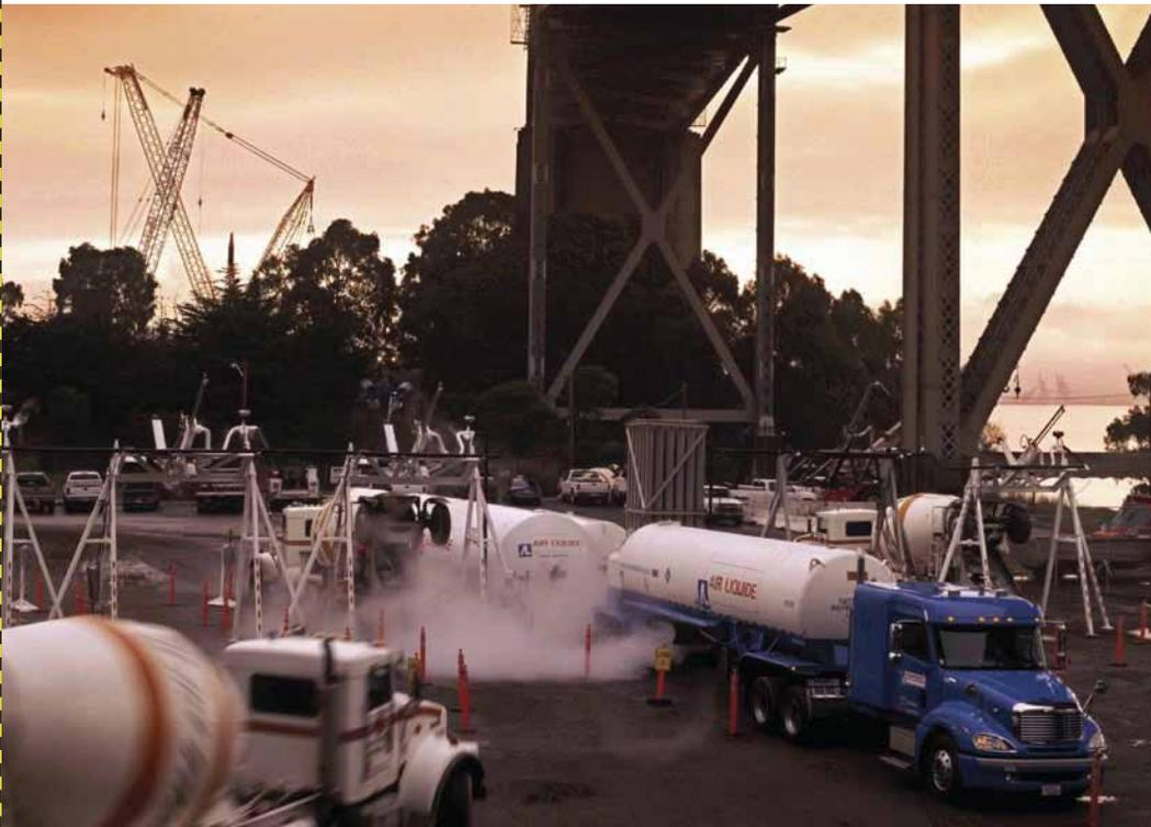
Concrete cooling with liquid nitrogen using Air Liquide's injection lance technology
